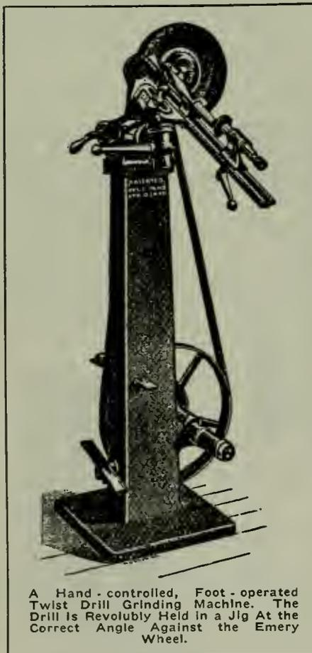
A Hand-controlled, Foot-operated Twist Drill Grinding Machine. The Drill is Revolvably Held in a Jig At the Correct Angle Against the Emery Wheel.
