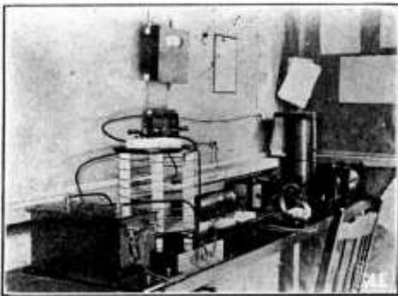
spark gap, glass plate condenser, helix, and hot wire ammeter. I use 110 A. C. with the coil.
