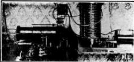
front of the loose coupler, electrolytic and silicon detectors, potentiometer and a pair of 4,000 ohm Holtzer Cabot phones.
